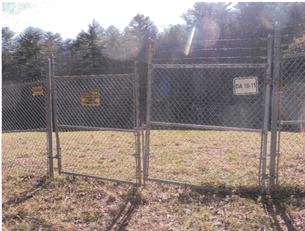
A locking gate and tall fence topped with barbed wire restrict access to FV disposal area DA-10/11. Warning signage is clearly posted on the fence that surrounds the cap.
