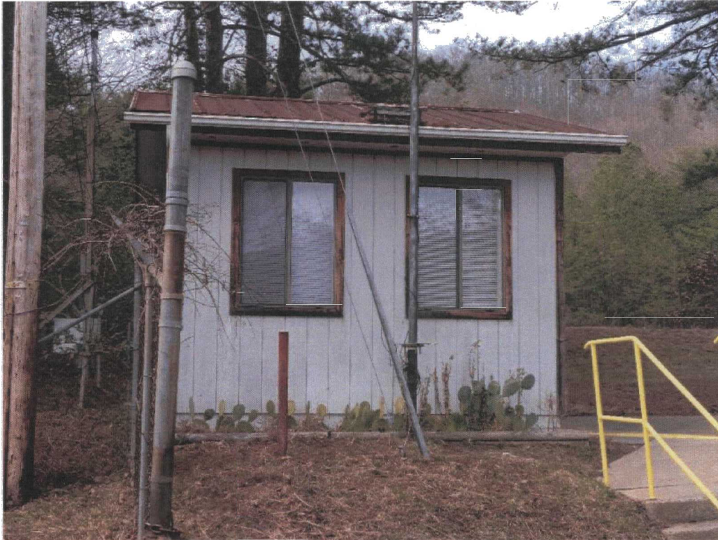
Upon site entry, all visitors must sign in with the security guard at this hut at the front gate.
