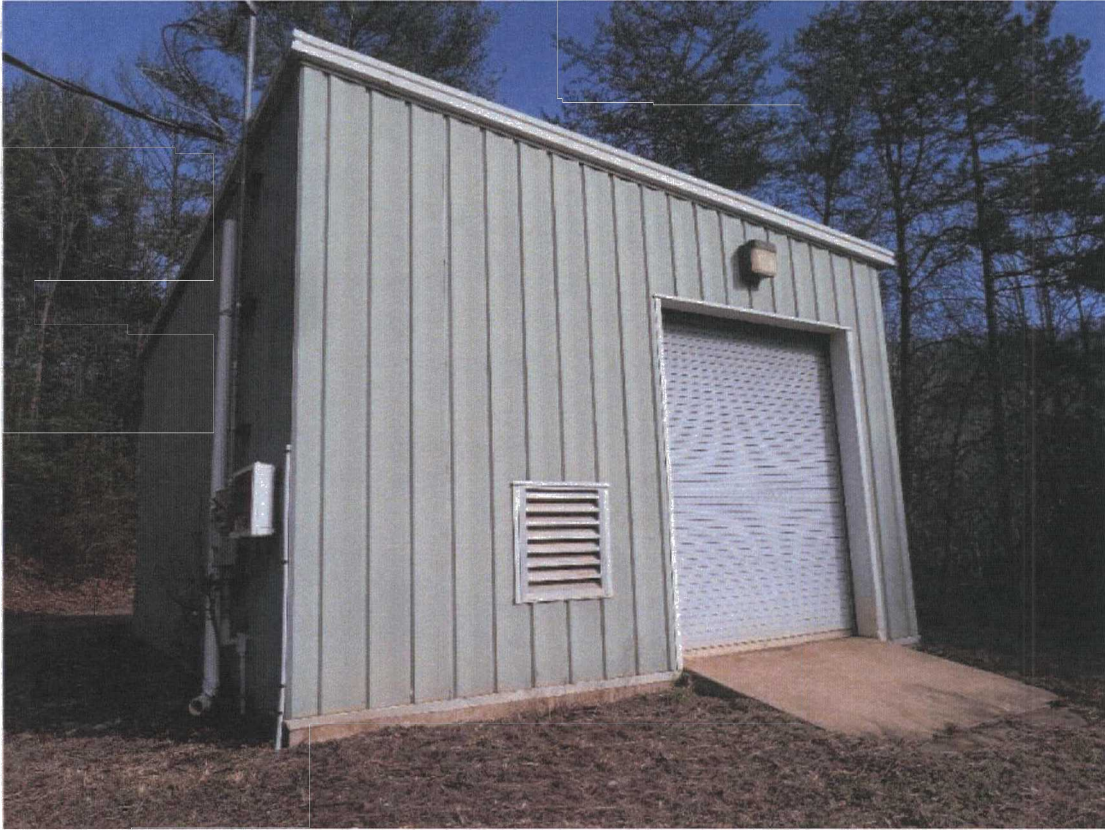
The BV groundwater treatment system is no longer in operation.
