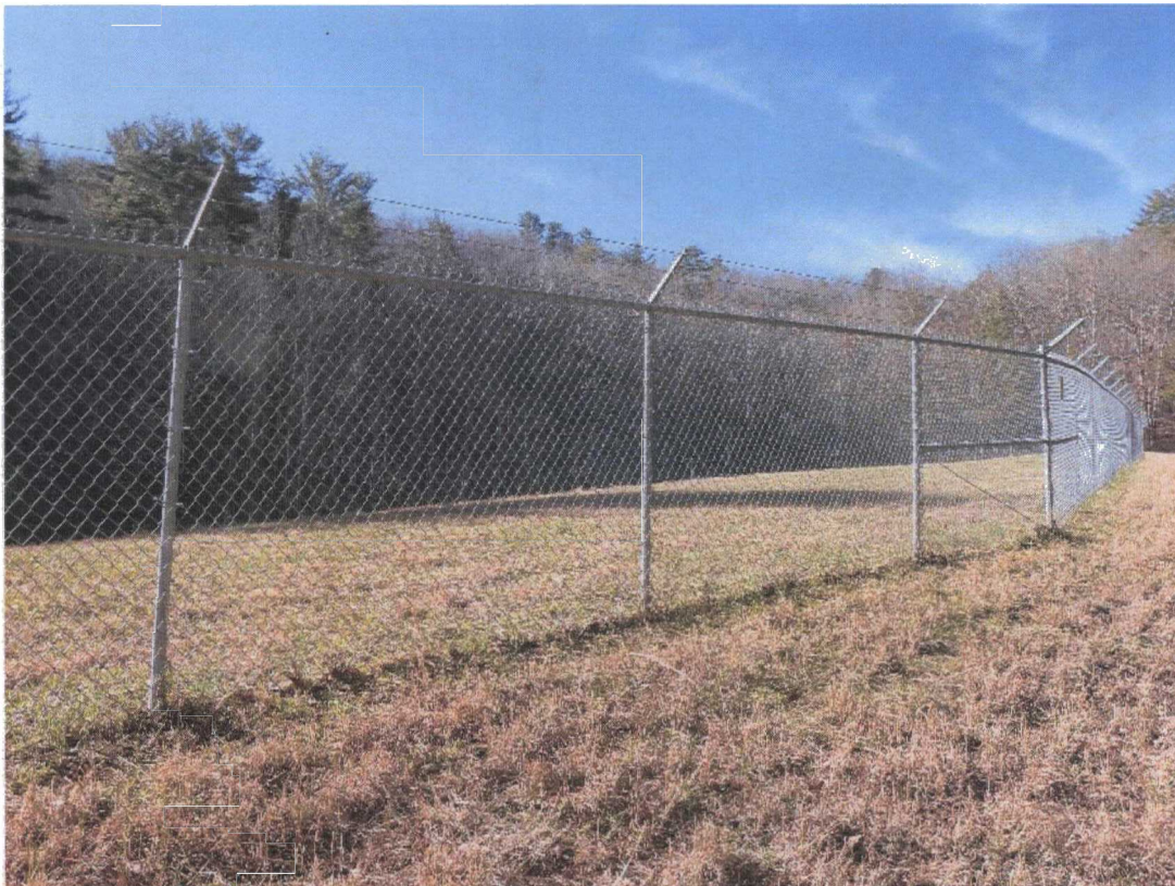
The fence that surrounds DA-10/11 appeared to be in good condition.
